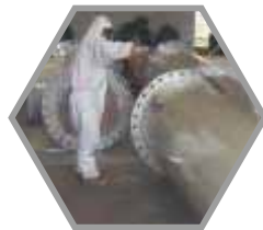
Structural Pipe Coating
